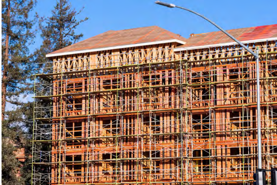
FIGURE 1 Multifamily residential building under construction in Santa Clara, California.
