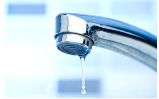
FIGURE 2 Leaks account for 16 percent of household indoor water use.
